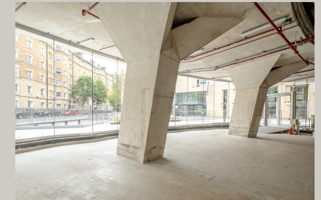
FILLING STATION | THE TOWER
